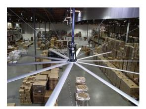
Figure 1-1: HVLS fan in industrial occupancy<sup>\*</sup>
