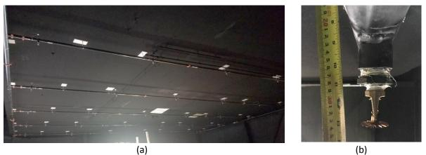
Figure 2-22: Sprinkler system (a) piping layout showing 10.2 cm (4 in.) cross main on left and 5.1 cm (2 in.) branchlines, (b) installed ceiling-level sprinkler.
