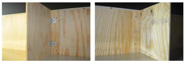
Figure 2-10: Construction of lateral flame break (penetrations at shelving upright covered by sheet of flame break material).
