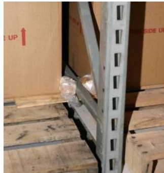
Figure 5-6: Igniter locations within the rack, located at the rack uprights
