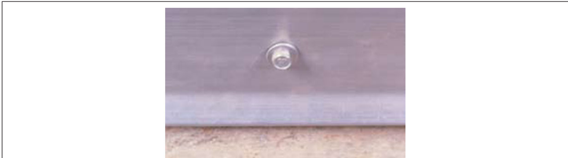
Fig. 2.3.2-1. Existing perimeter flashing secured at its lower edge
